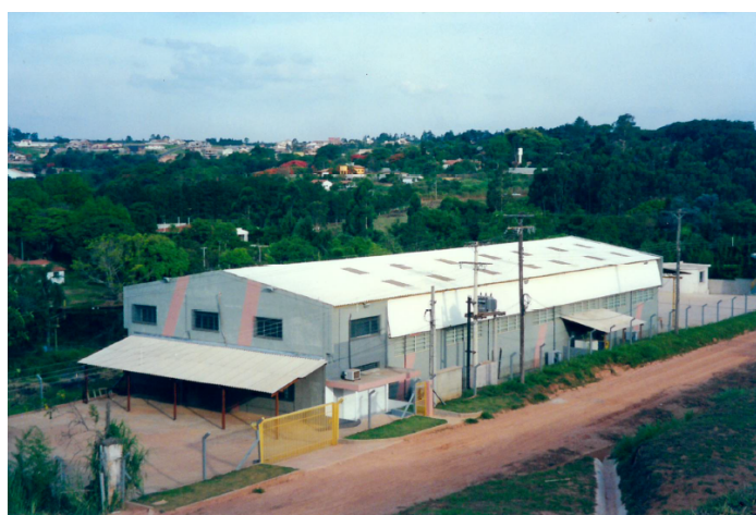
(2) First production plant in 1999.
