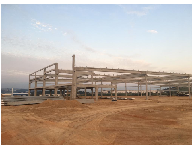
(15) Land for the new building in Vinhedo.
