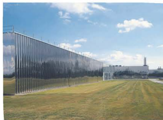
Aplix S.A - Headquarters FRANCE - 1 factory
